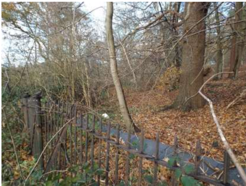
A glimpse over the railings shows the line of the road leading off into the woods. Over the years there have been occasions when some car drivers have mistakenly ventured down the old route, flattening the fence on the way.
