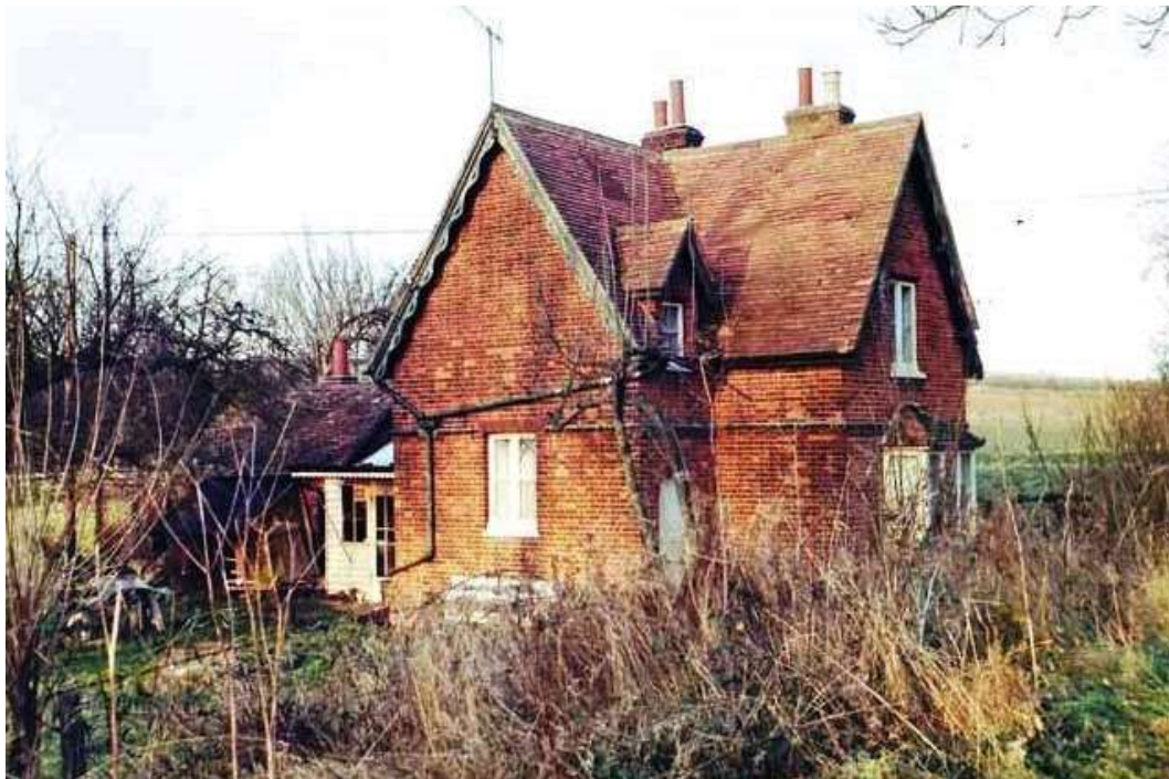
A 1983 view of the railway crossing keeper's cottage.
